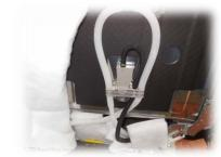
Most dishwashers do not have built-in backflow prevention from the drain hose
